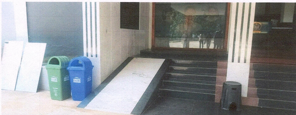
Ramp at Civil Engineering Block
