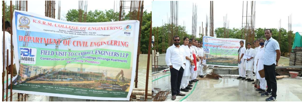
Fig. G+4 Construction site visit by V sem B.Tech., Civil Engineering students and Dr. N Amaranatha Reddy, HoD CE.
