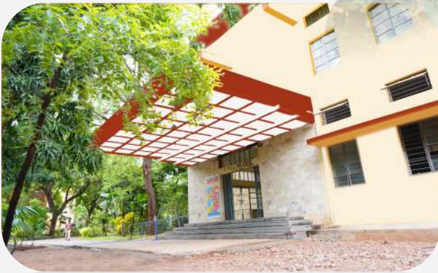
Civil Engineering Block
