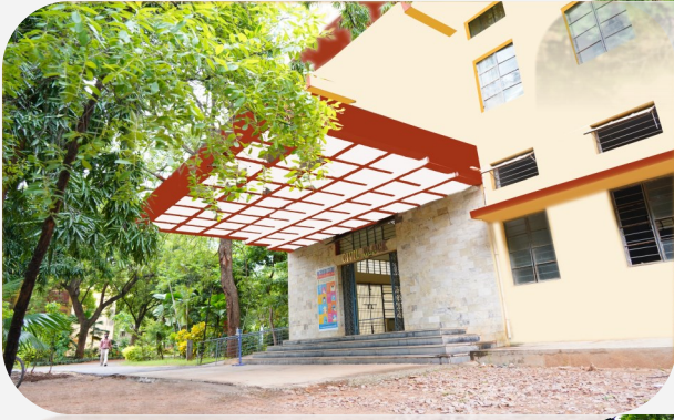
Civil Engineering Block
