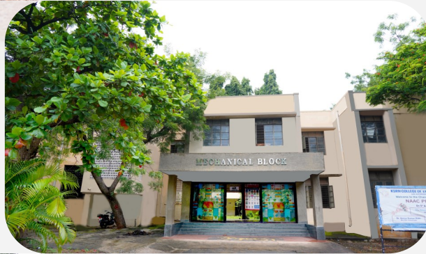
Mechanical Engineering Block
