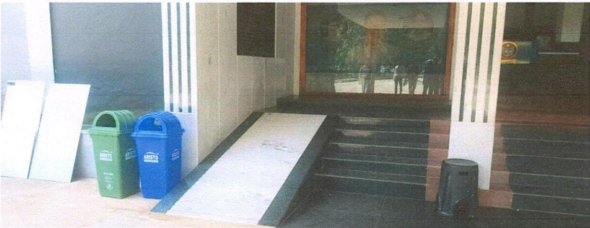
Ramp at Civil Engineering Block
